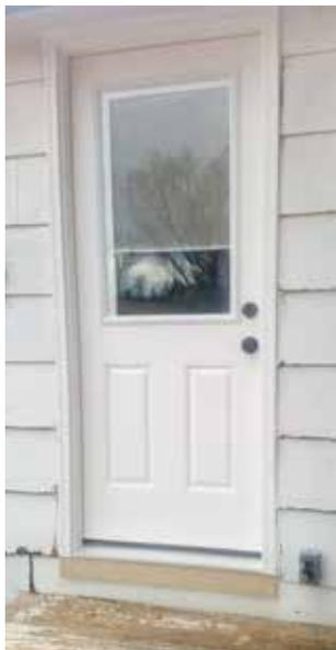
Right: The front and back doors of Sharon's home were replaced with insulated doors and new weather stripping that will reduce drafts and energy loss.
